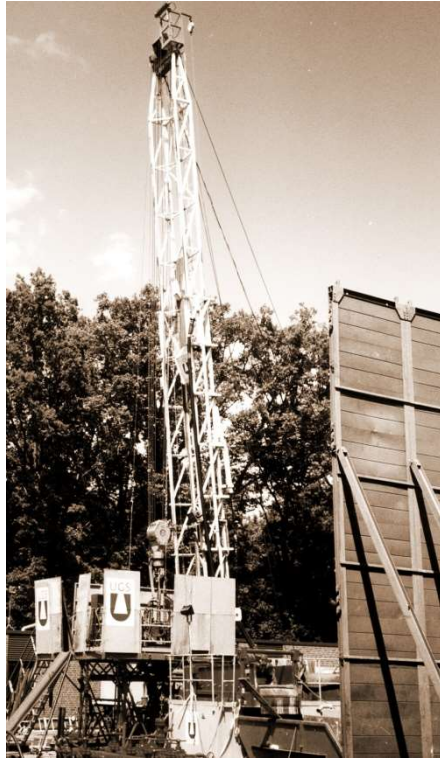
The Franks 200 workover rig in operation, combined with a noise wall.
